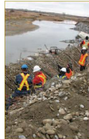
Students install willow branches (left) and TRM & Scour Stop (right).
